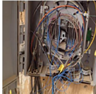
*Poor installation becomes worse over time and faults accumulate. A typical installation is shown here. The low IP rating of the components also contributes to this high fault rate. Hardened connectors would avoid this problem.*
